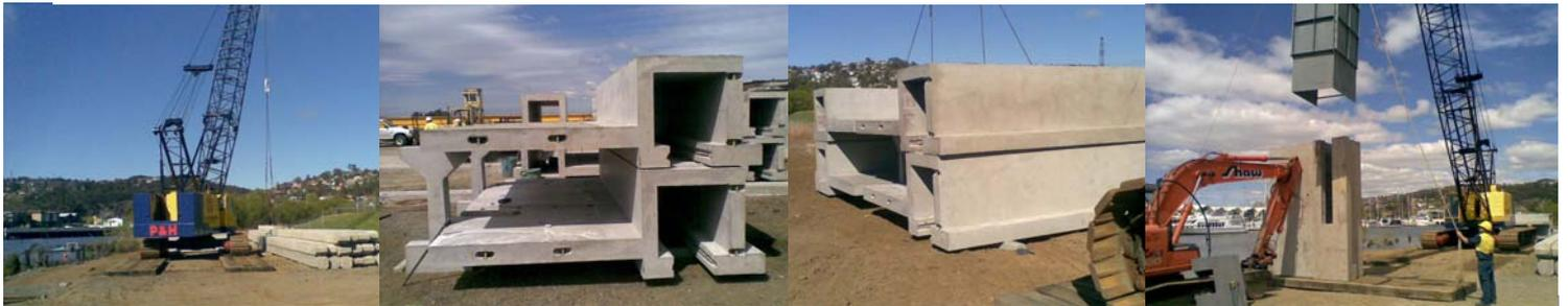
Hayward's 150 tonne crane lifts the 18m piles from the storage area to the PLA barge for driving. Each wall section is then lowered over the two (vertical and raked) piles. The wall panels are being cast at our new Western Junction facility near Launceston Airport.
