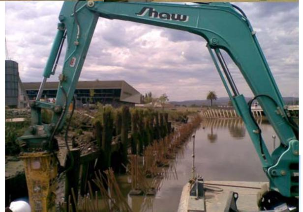
Once the piles have been driven and broken down to the correct height, a wall panel (shown with a protective work box attached) is lowered into place. These photos show the 'special' starting panel being installed and the finished product after forming and pouring. Note the tops of the piles are visible (at right) for 30 minutes at low tide only.
