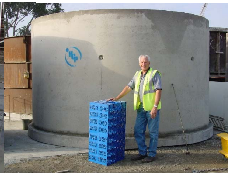
Roxley once again with a Raincell detention unit standing in front of a 4m Dia, 25,000 litre detention tank.
