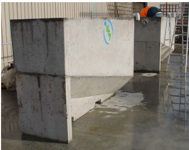
Roxley (supposed desk job) fitting out our new Grease trap and Triple Interceptors.
