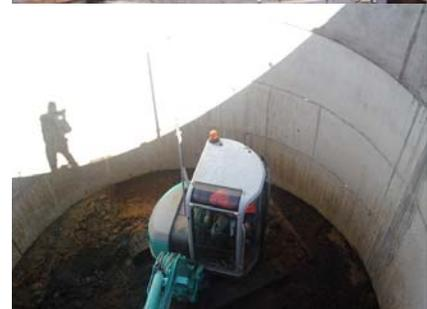
As the shaft sank further sections were added and all joints were grouted and sealed above the ground. All went well and the caisson progressed in textbook style to a point about 500mm above its final position. Sinking was delayed until a number of arrestor pad footings were poured under the shaft to ensure that it stopped in the final position.
