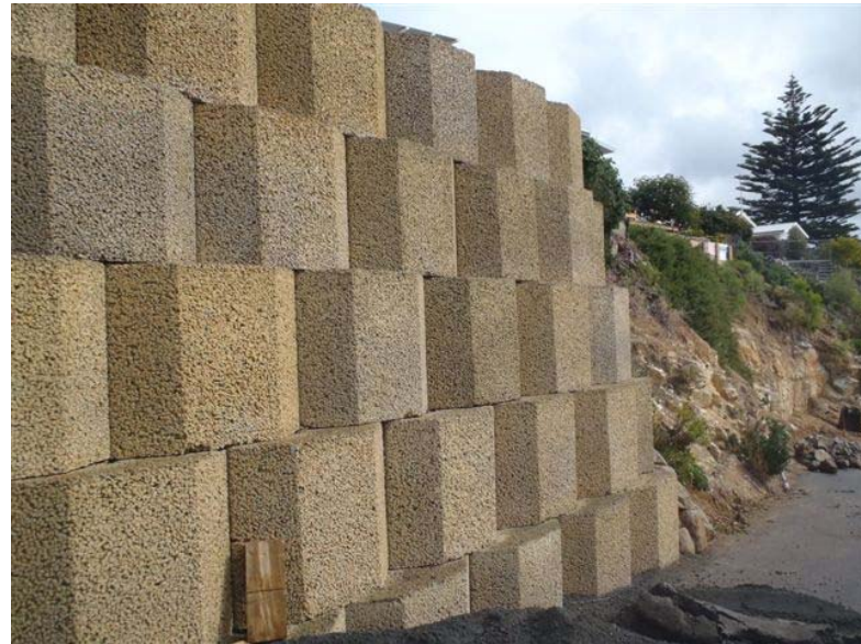
SANDSTONE MASSBLOC WALL
