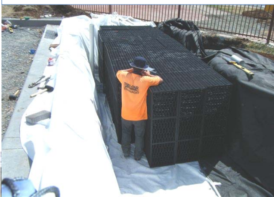
250 KL Detention tank, Flushable modules
